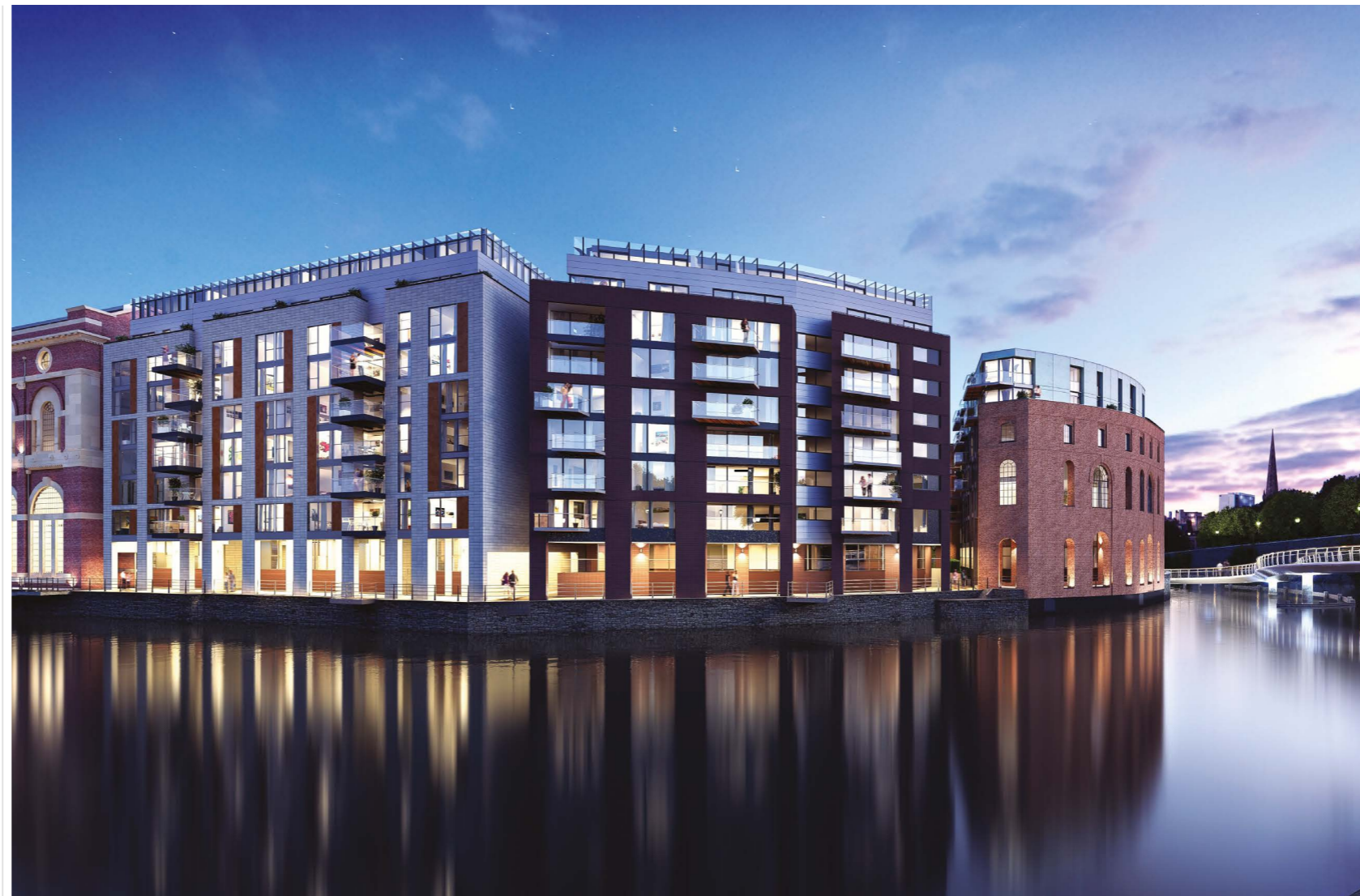
Opposite and below: Finzels Reach in Bristol is a major build-to-rent development that Willmott Dixon is building for local developer Cubex, on behalf of Grainger.
