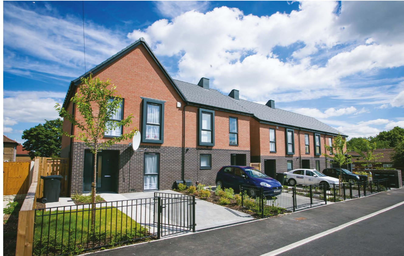
Below: New homes at Trent Basin in Nottingham. Opposite: Willmott Dixon has built more than 100 new homes in Doncaster that cater for all tenures.
