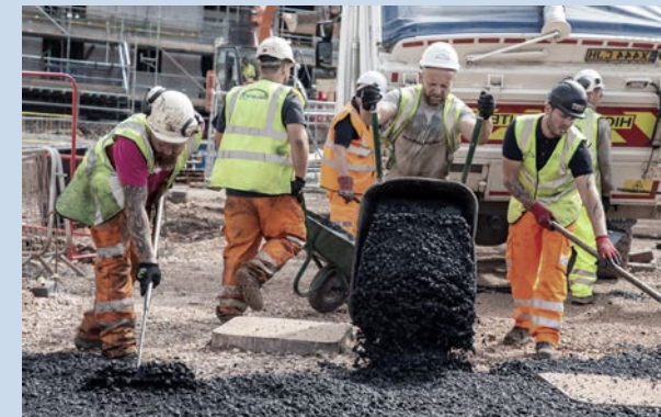
▼ Green asphalt at Ashton Rise, Bristol
