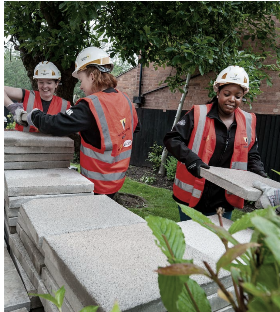
▼ Renovating a Salvation Army Housing Association training facility
