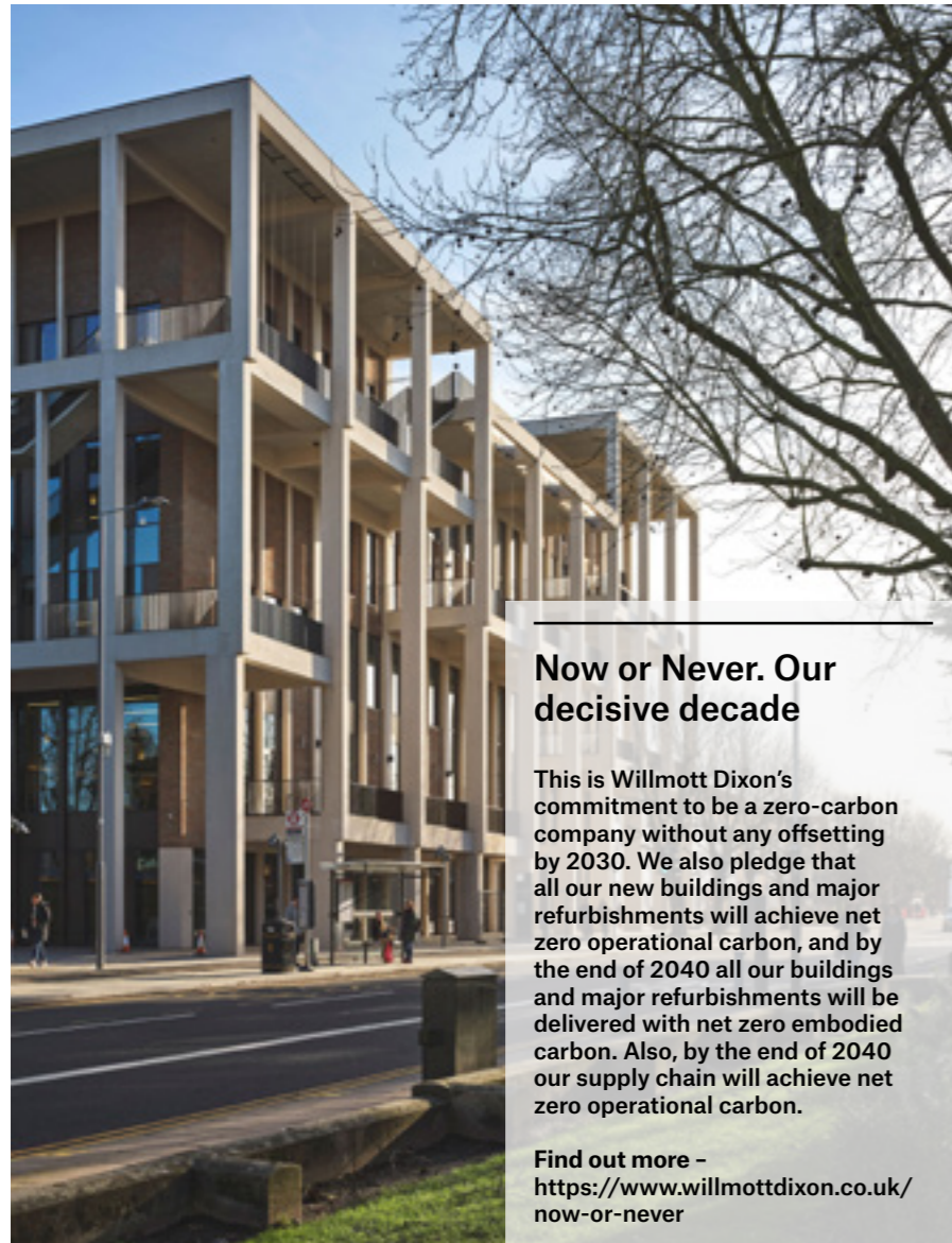
Left: The 2021 Stirling Prize-winning Town House for Kingston University used a specially formulated concrete with lower embodied carbon.
