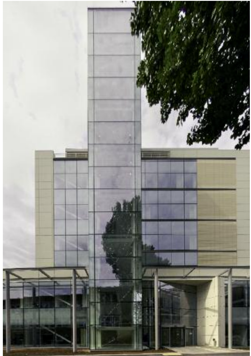
The Institute of Life Science, one of Europe's foremost facilities to research life sciences, built for the University of Swansea.
